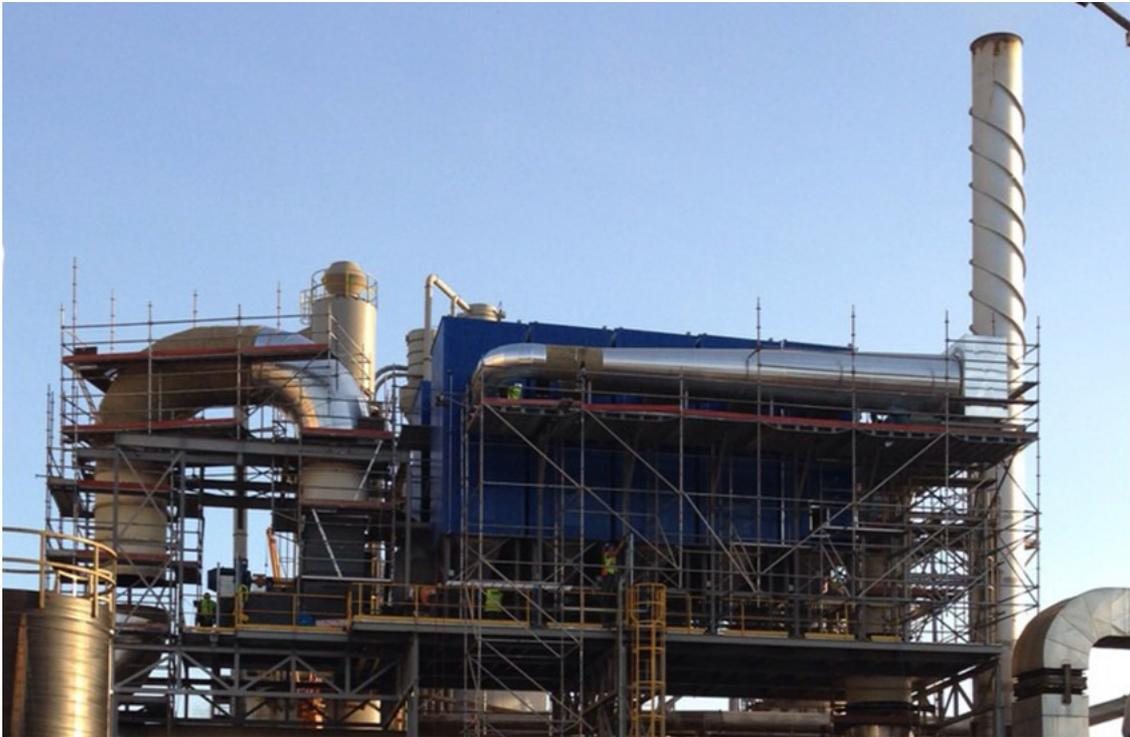
**Hurricane® HR** cyclone system (10 batteries of 6 cyclones) to reduce PM emissions, including unburnt carbon particles from a 40MW<sub>th</sub> wood waste boiler operating at 247 088 m<sup>3</sup>/h at 303°C.
